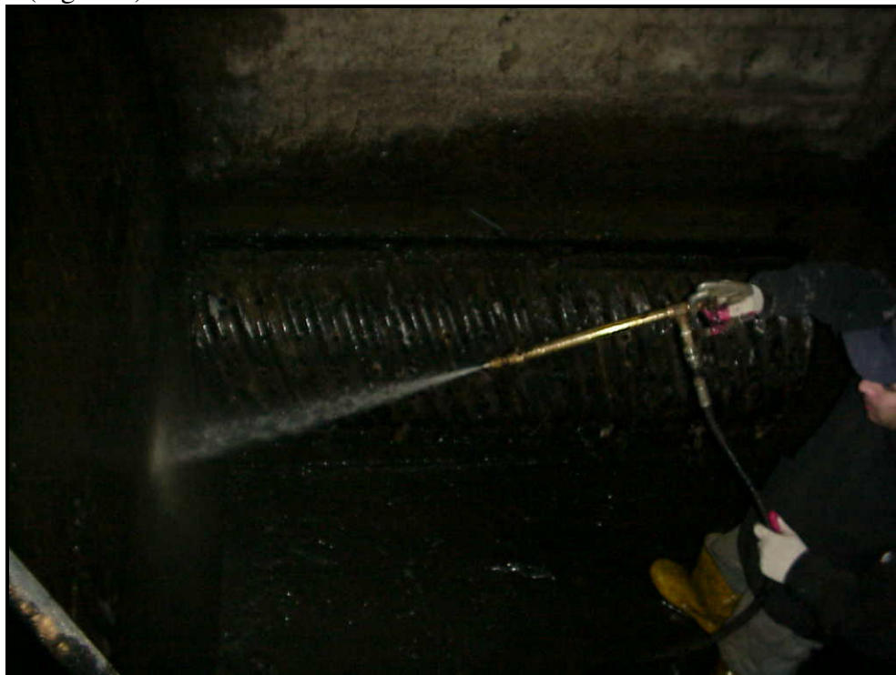
Figure 1. Manual access to every chamber of a manufactured BMP was deemed critical. (Photo courtesy of Richard Gee, Montgomery County, MD.)
