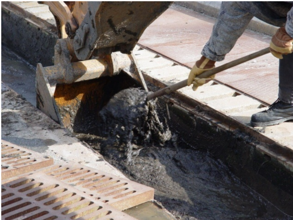
Figure 4. Harvested materials (in this case from a Delaware Style Sand Filter) must be disposed of in a safe manner. Placement in the appropriate type of landfill is recommended. (Photo courtesy of William Hunt, NC State University.)
